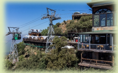
Harties Cable Way
