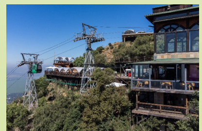
Harties Cable Way
