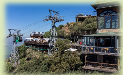
Harties Cable Way
