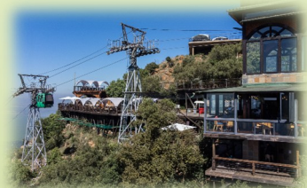
Harties Cable Way
