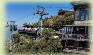
Harties Cable Way
