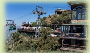
Harties Cable Way
